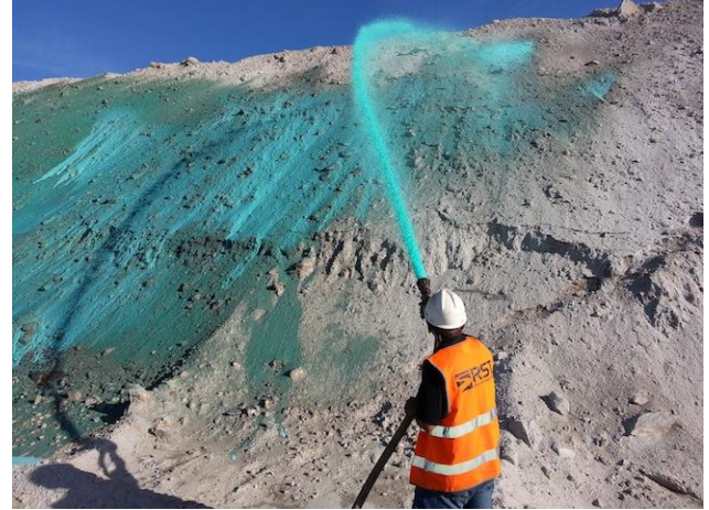
Figure 2. Soil binder and mulch application prior to rain
