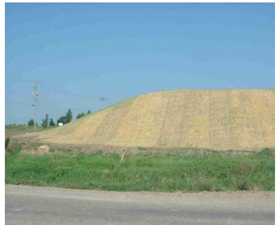
Figure 4. Stockpile stabilized with erosion control blanket
