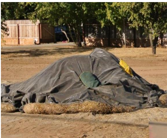
Figure 5. Contaminated stockpile under cover
